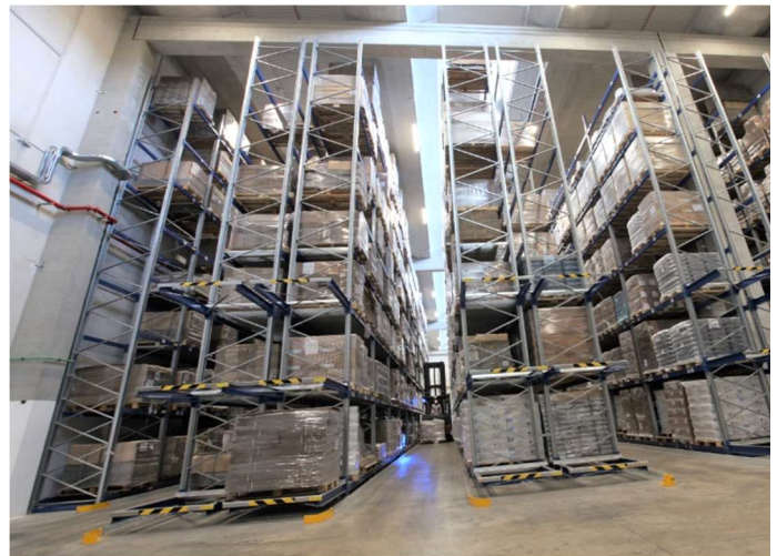
The new central warehouse
