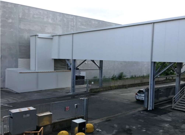
The Tunnel connecting the new central warehouse to production
