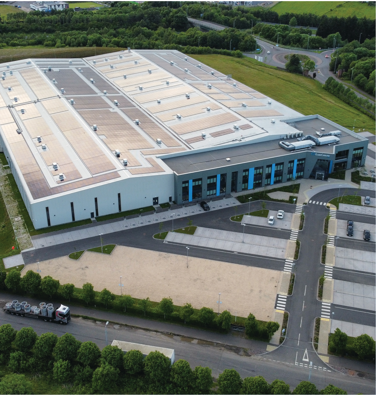
Guala Closures, an independently managed company of Investindustrial Fund VII LP, has integrated 2.4 MW of rooftop solar panels in its newly developed Gartcosh facility in the United Kingdom. This facility is strategically located in Scotland's whisky-producing area, serving both major global brands and smaller producers.
