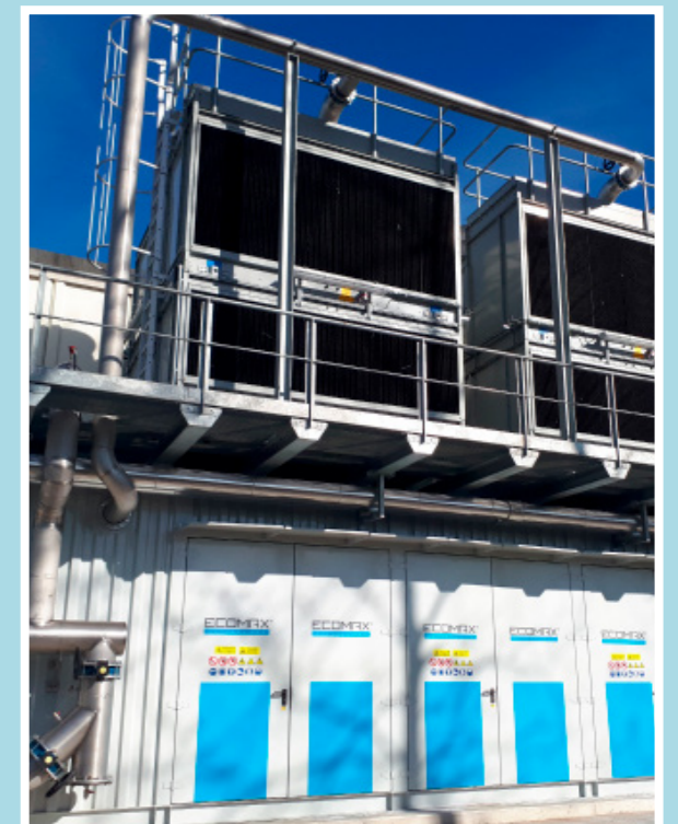
MTD is developing a trigeneration plant similar to Artsana plant, as pictured.
