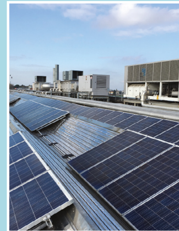
Sergio Rossi's photovoltaic system installed at its San Mauro Pascoli plant in Italy.
