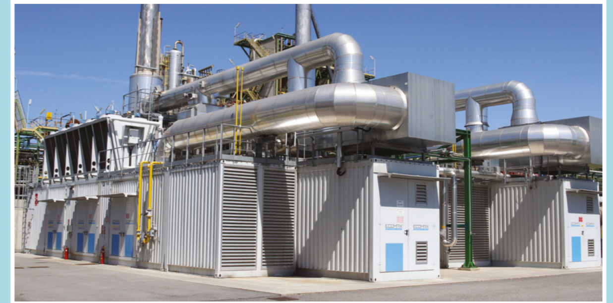
The co-generation plant at Polynt Reichhold's Scanzorosciate site in Italy.
