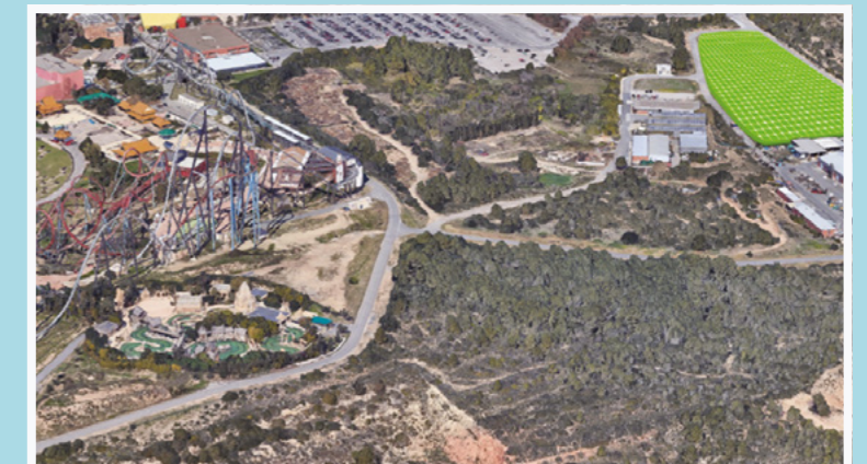
PortAventura World's photovoltaic plant will cover 89,000 square metres, or roughly the size of 14 football fields and will be the largest in a European resort.
